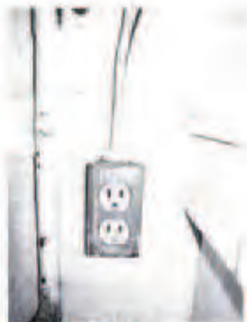
Photo 15 improper wiring
