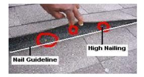
**Note:** *Jumbo and some premium shingles* have a different measurement, so be sure to check the installation instructions for correct placement of the nails.
