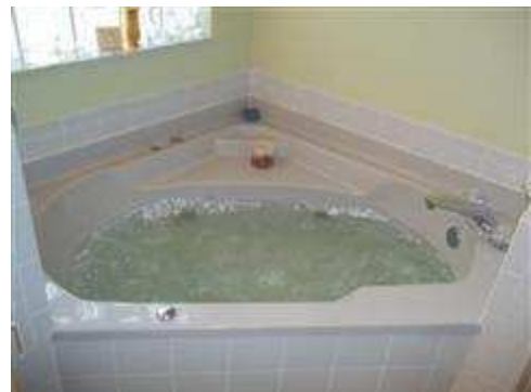
Hot tub being tested.
