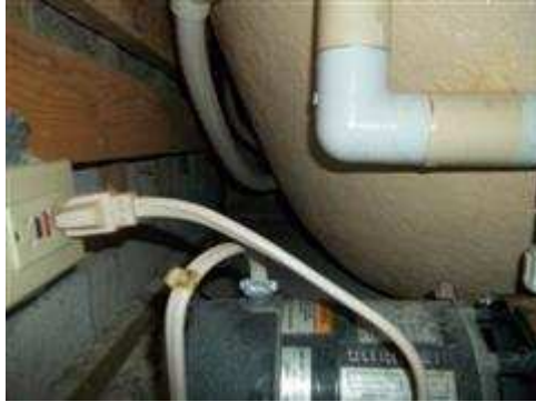
Area under hot tub.
