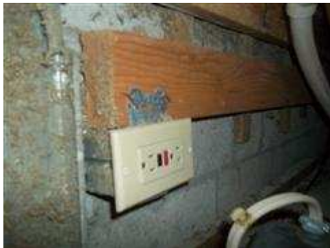
G. F. I. receptacle did not trip when the test button was pressed under the hot tub.
