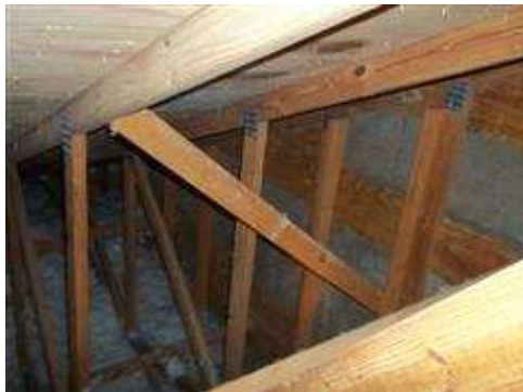
Attic gable end.
