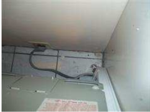
Anti-tip bracket was not present at range.
