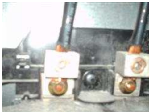
Main lugs and wiring in kitchen panel.
