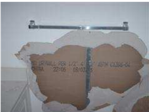
Chinese drywall observed in upstairs rear bathroom,.
