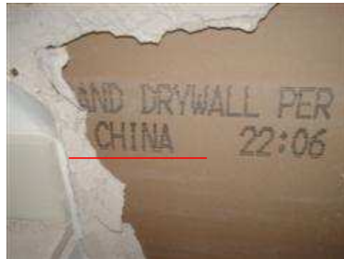
Chinese drywall observed in upstairs rear bathroom,.
