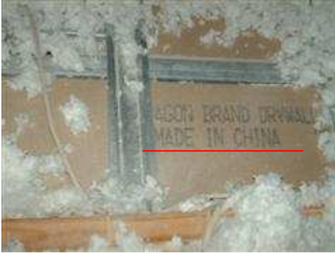
Chinese drywall observed in attic.
