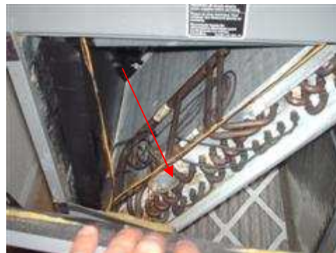
Air handler coils were corroded.
