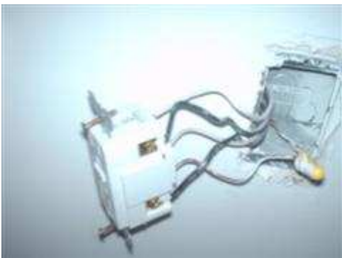
G.F.I. receptacle wiring observed in downstairs bathroom.
