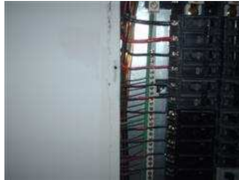
Copper ground wires observed in kitchen breaker panel.
