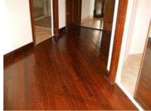
The flooring in the master bedroom was damaged from an apparent water leak, possibly from the air handler.
