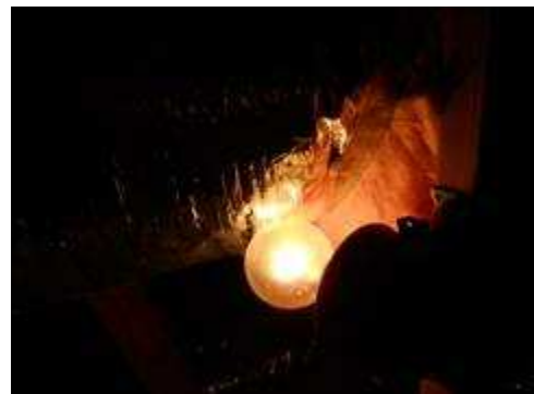
Duct line above master bedroom closet is directly over the attic light fixture.
