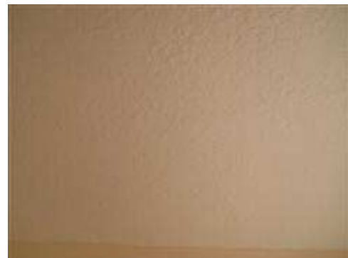
. There was only one form of ventilation present in the addition bathroom and two are required.
