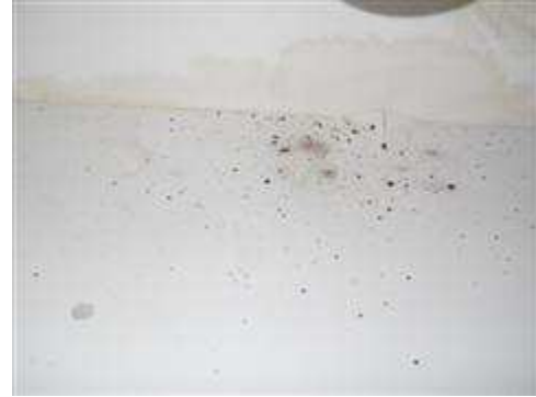
Vanity in upstairs bathroom was damaged.
