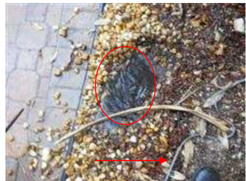
Exposed wiring observed in numerous areas of the yard for the landscape lighting. Several sprinkler heads were not present.
