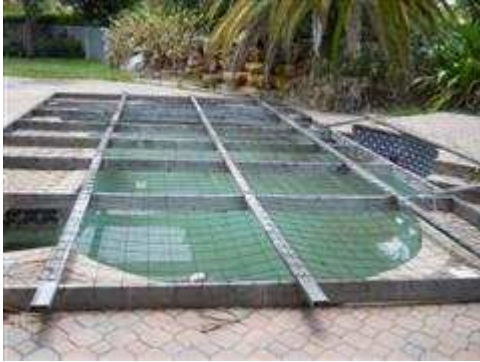
The swimming pool was not in a condition where it could be inspected.
